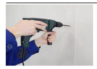
2. Drill holes for chosen fixing system.
