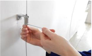
7. Secure the cable in tightener by tightening bottom screw, remember to leave some clearance for correct functioning
