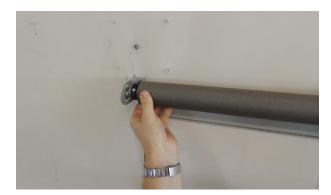
7. Slide the roller tube to the bracket on motor side.
