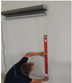
3. With spirit level mark places for cable guide bracket installation.
