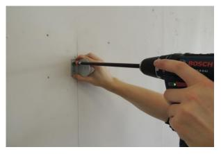
4. Mark places for holes and install second bracket to the wall/ceiling.
