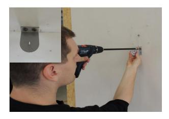
3. Install first bracket to the wall/ceiling, adjust if necessary.
