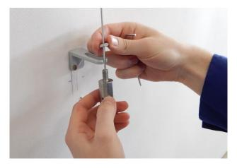
6. Install façade tightener to the bracket.
