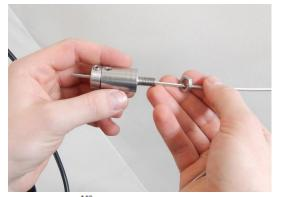
5. Put cable through façade tightener.
