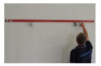
5. Check vertical and horizontal levels, correct if necessary.
